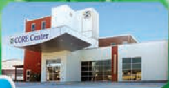
New downtown Washington $5 million orthopedic healthcare expansion (main Daviss Community Hospital operations managed by St. Vincent - one mile west)
