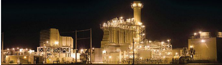
Idaho Power's new 300 MW power plant operating with natural gas and steam turbines joins their hydro and wind portfolio
