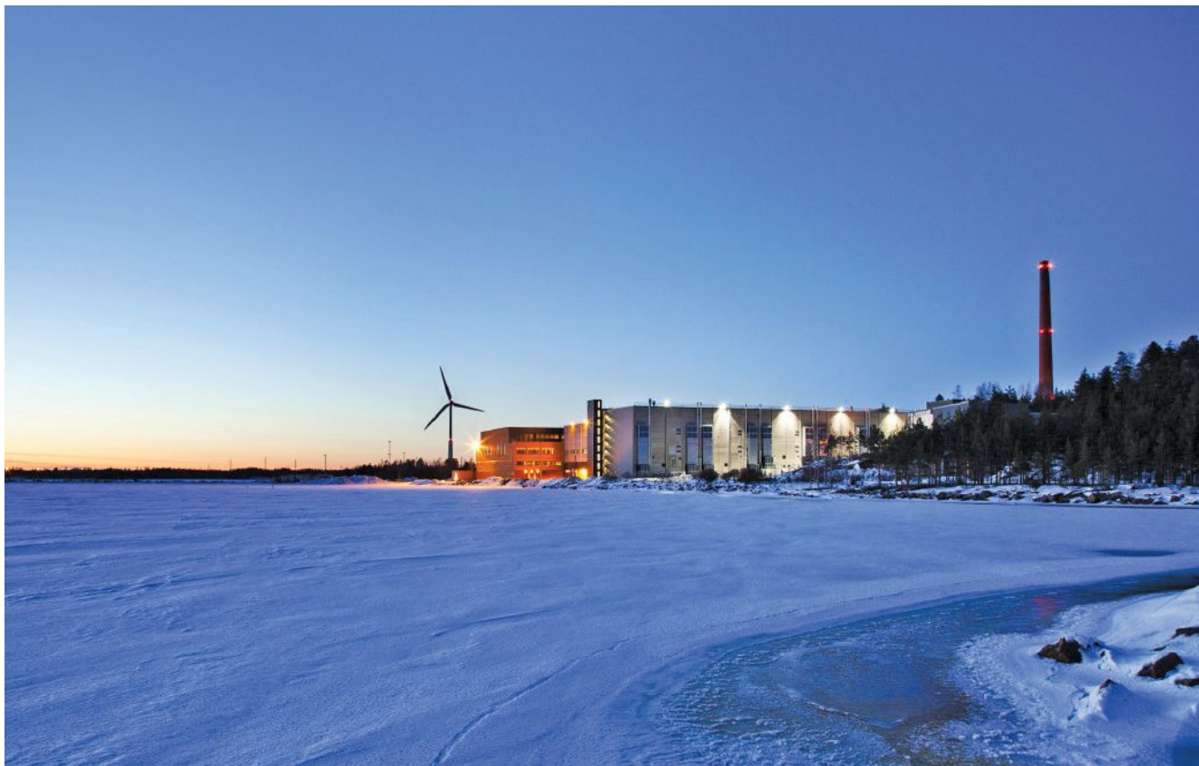
Located on the shores of the Gulf of Finland, this Google data center in Hamina, Finland, is one of seven large data centers that Google owns and operates outside the U.S. Photo courtesy of Google
